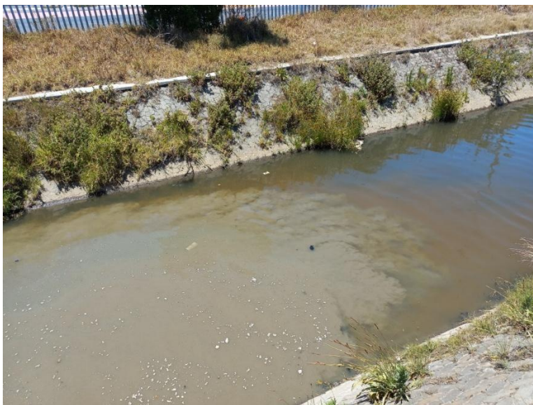
Photograph 5.2.1. Spill from the surcharging Koeberg Pump Station
