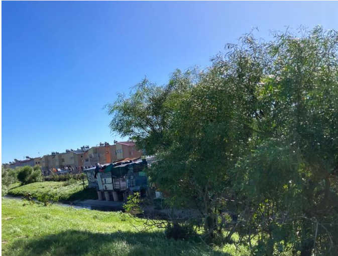
Photo 8.4.1 Informal housing built right over the edge of the Jakkalsvlei Canal, along the N2 past Langa
