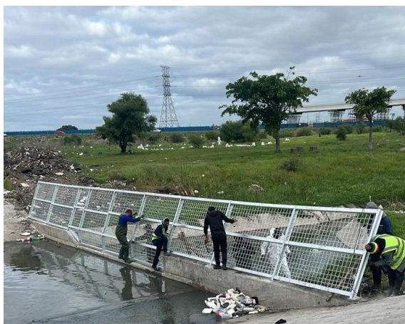
Photo 8.8.5 Newly constructed litter fence on the Big Lotus River (one of five litter fences as of June 2025). Photo: CSRМ
