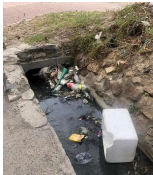
Photo 8.6.4 Litter blocking a stormwater drain in Imizamo Yethu [image from Lukhozi 2023]
