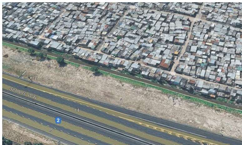
Photo 8.4.2 November 2024 Google Earth image of Langa informal settlement, showing shack dwellings abutting and overhanging the Jakkalsvlei Canal
